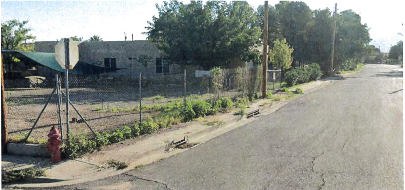
Appendix Image 12. Many of the sidewalks in the Mesquite area are not ADA accessible and create a barrier to universal access throughout the neighborhood.
