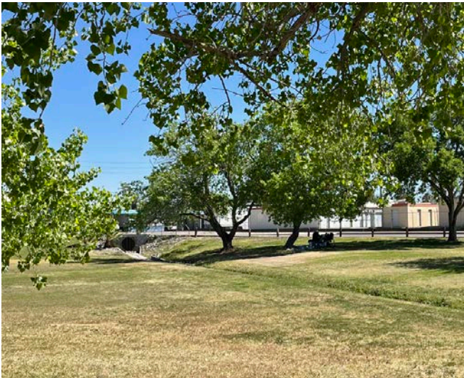
Frenger Park's stormwater infrastructure.
