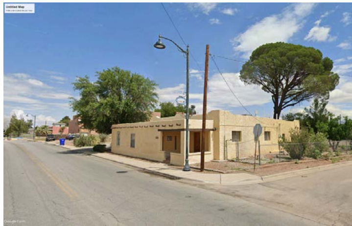
One of the many historic adobe structures in the neighborhood.
