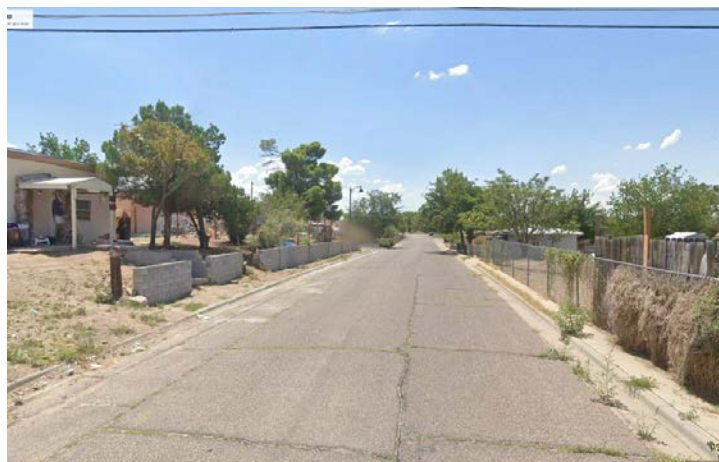
Some streets lack pedestrian facilities, but traffic is low so they likely function as “shared streets”.
