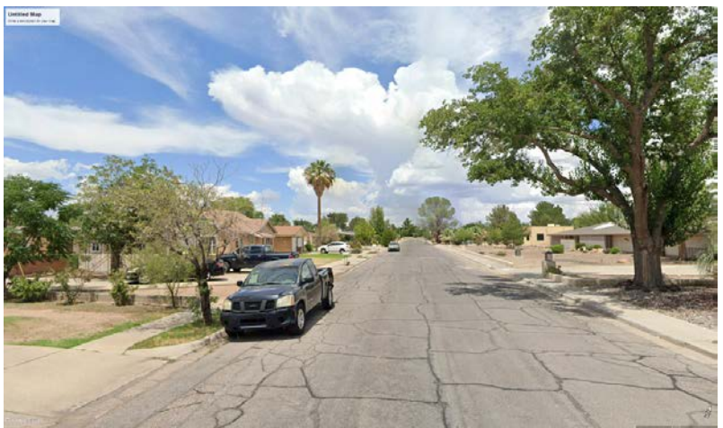
View along Turrentine Drive.
