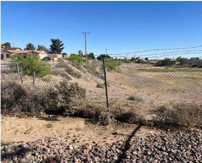
Stormwater retention area next to Valley View Park.
