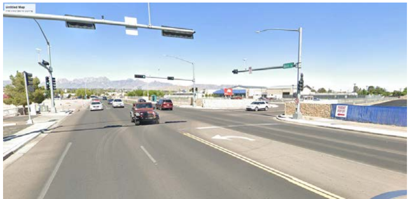
Vehicular entry to high school on Boutz Rd.
