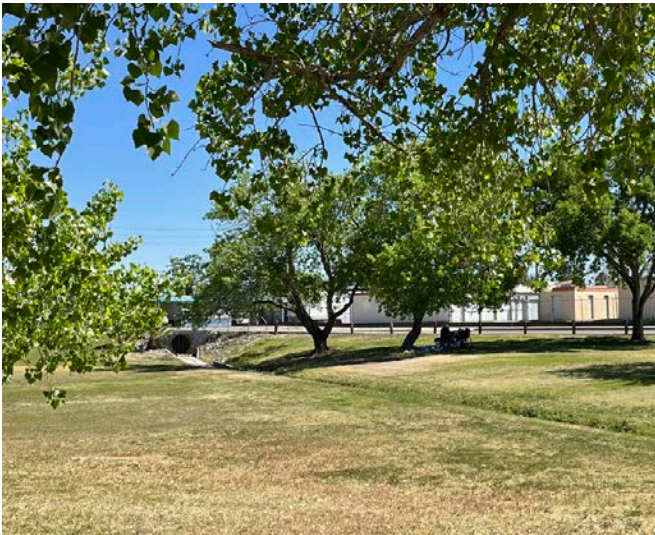
Frenger Park's stormwater infrastructure.
