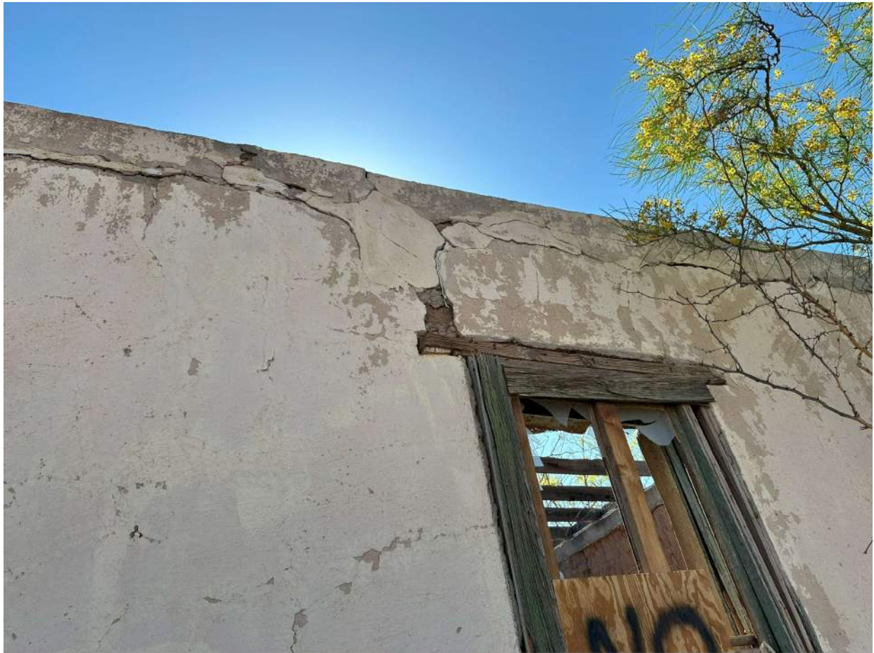
Photo 6 West side of west unit
