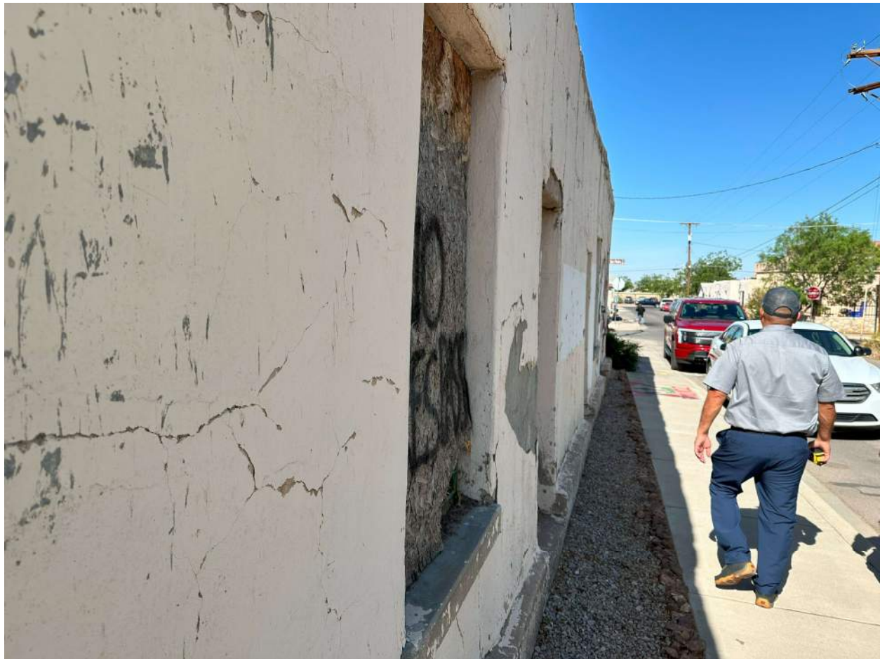
Photo 5 Front of west unit.
