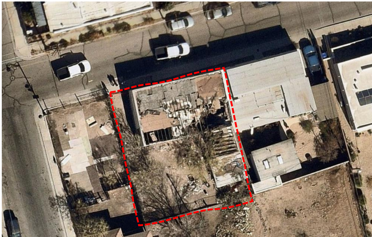
Figure 1: Aerial of property at 414 E. May, with property boundary highlighted in red. Aerial was taken on February 7, 2025, and collected from Nearmap. The south wall has not collapsed in the photo, suggesting that the collapse has happened in the months following February 2025.
