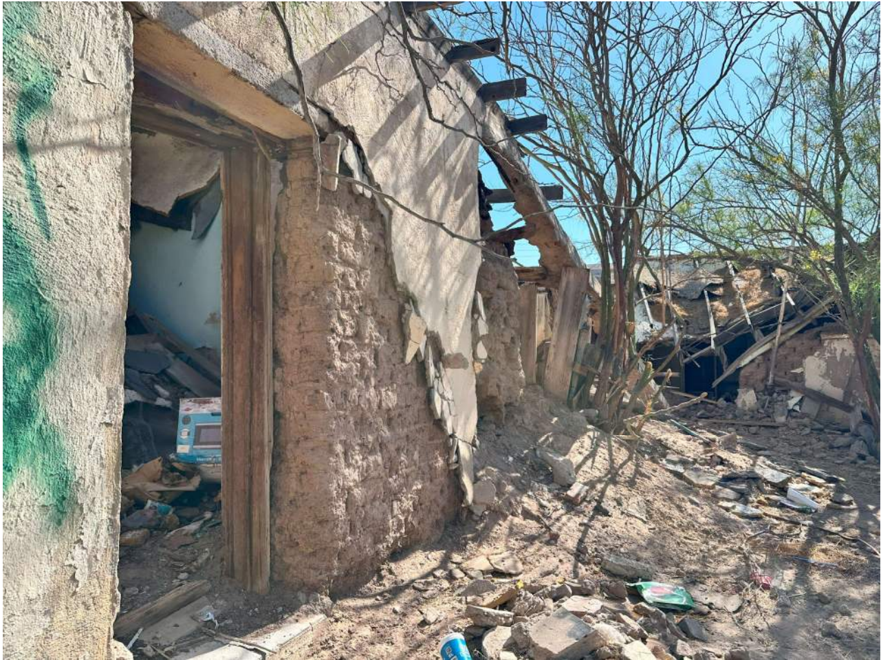
Photo 7 Rear of west unit
