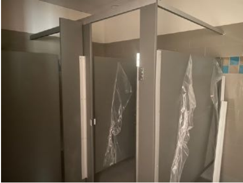
Newly Renovated Office Wing – Restrooms
