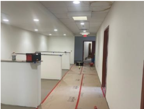
Newly Renovated Office Wing – Office Cubicles
