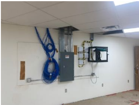
Newly Renovated Office Wing – Electrical / IT
