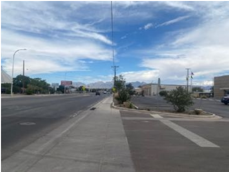
Street view east of Amador Ave.
