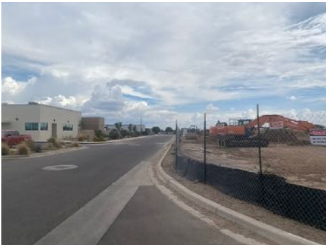
East north to south interior access road.
