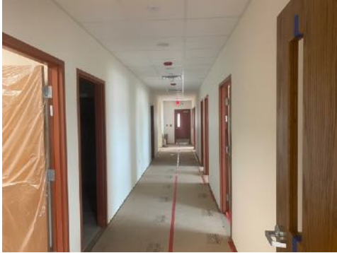
Newly Renovated Office Wing – Interior Corridor
