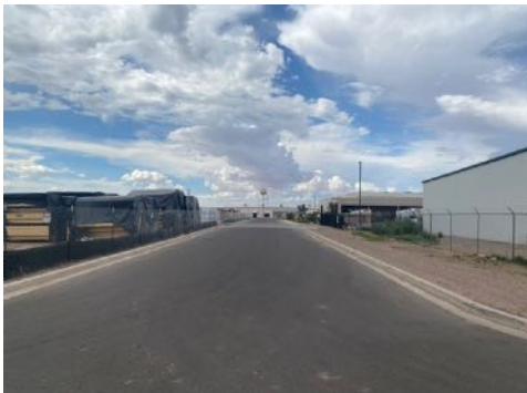
Eastern south to north interior access road.
