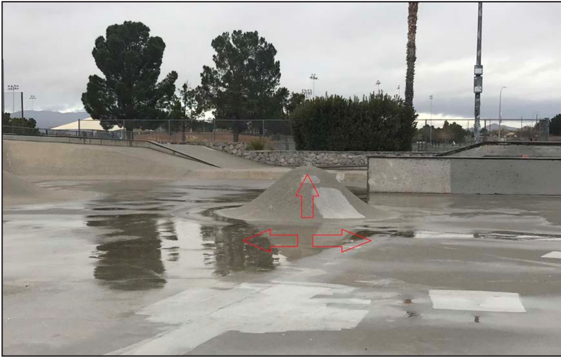
Feature #17 (low speed) - Pump Bump: This feature is in a good location within the skatepark design but it is too steep and not long enough.
