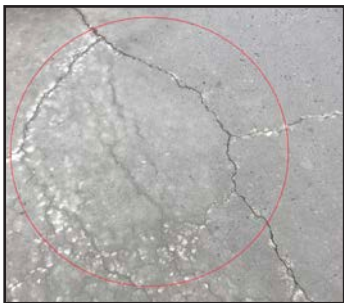
Spalling/Cracking
