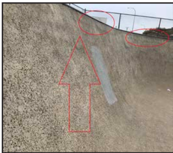
Exposed Aggregate/ Steep Transition
