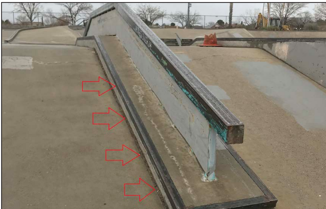
Feature #9 (low speed) - Kinked Grind Rail: This rail is good in height but it sits on top of another ledge type of obstacle that could be hazardous when trying to ride the rail. Typically a grind rail is fastened independently into the concrete. The ledge underneath the grind rail has potential to be a tripping hazard.
