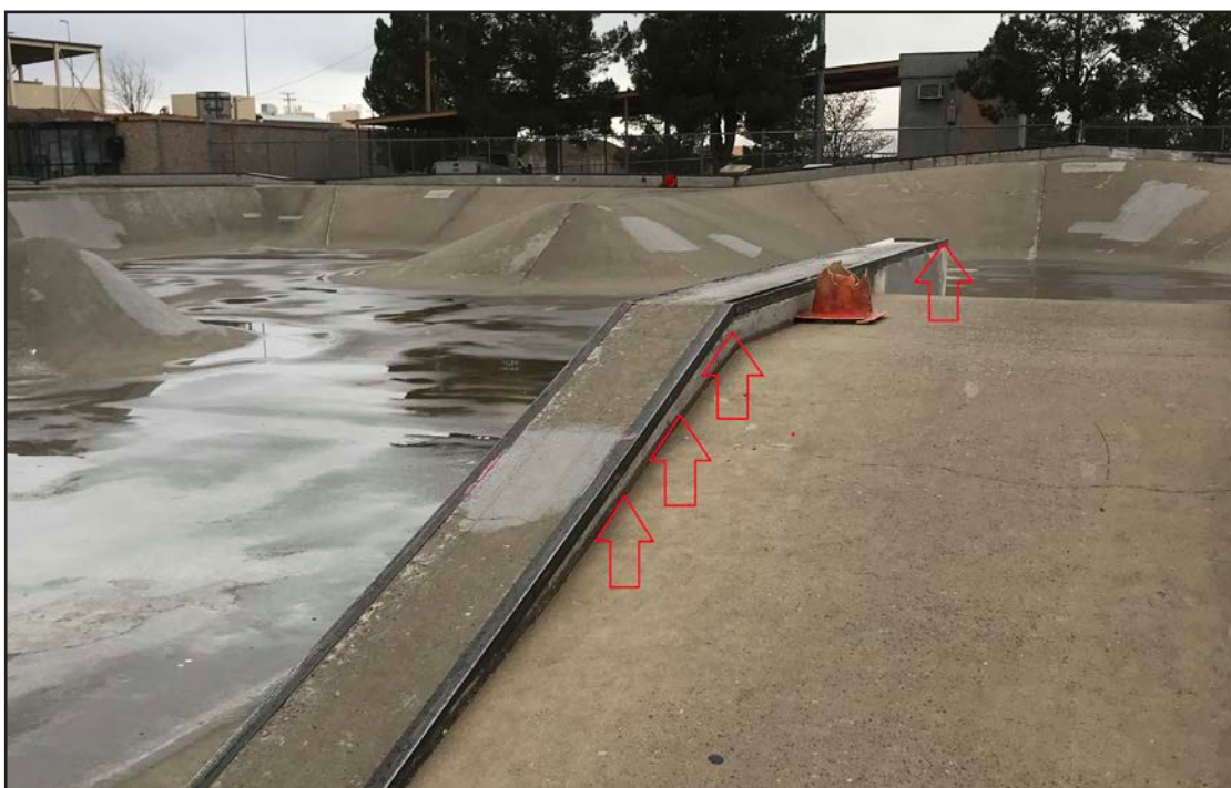
Feature #10 (low speed) - Straight Ledge: This ledge is relatively low in height for how tall the approach ramp is. The end of this ledge drops straight to flat, which is okay but not preferred as the ledge height at the end is very high.
