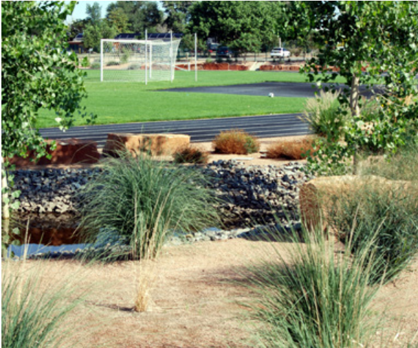
Low Impact development feature, bioswale
