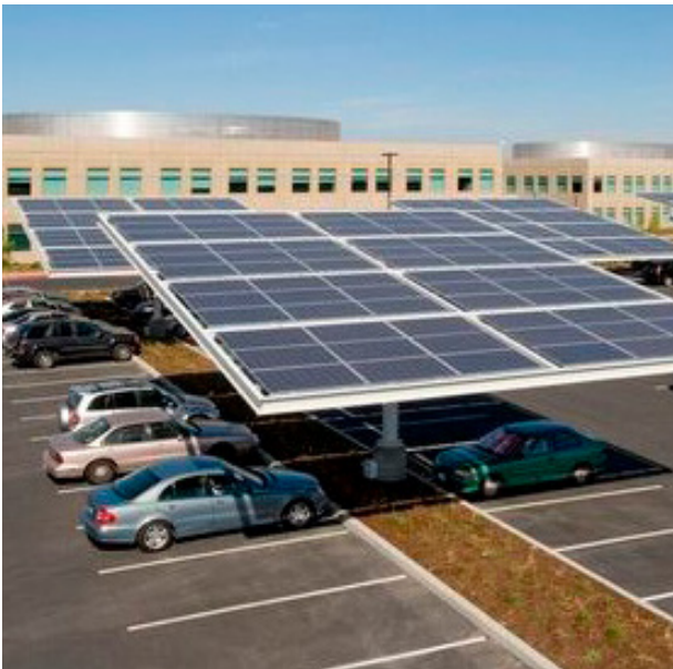
Energy production through Solar covered parking lots
