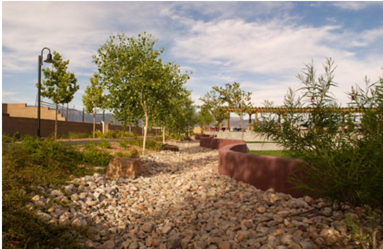
Low Impact development feature, bioswale
