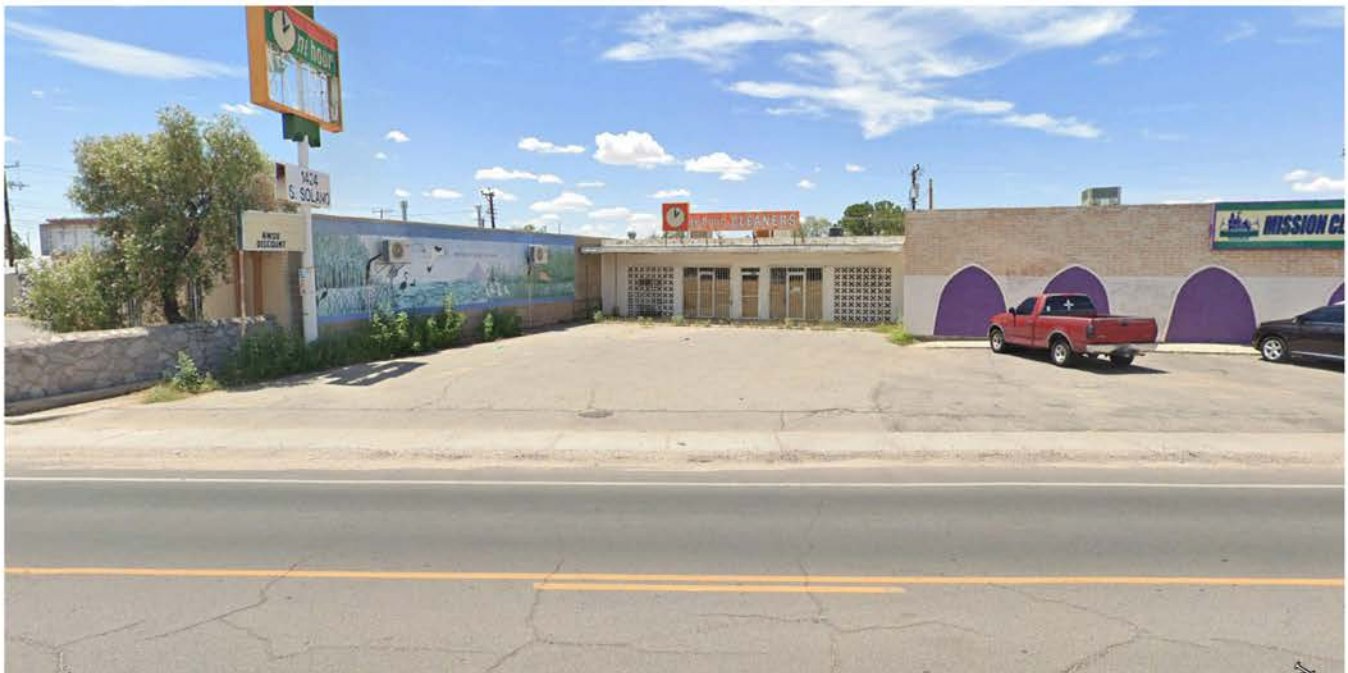
Image 5. Abandoned dry cleaners, boarded up windows and outdated signage could discourage new investment along the El Paseo & South Solano corridors.
