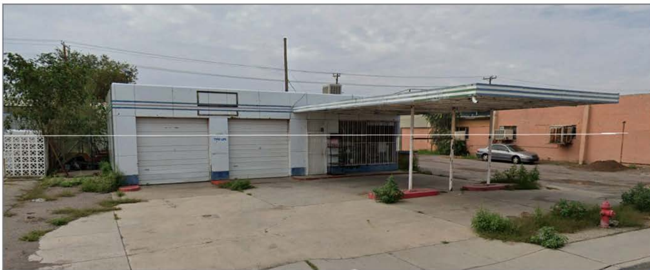
Image 20. Vacant gas station on West Picacho Ave.
