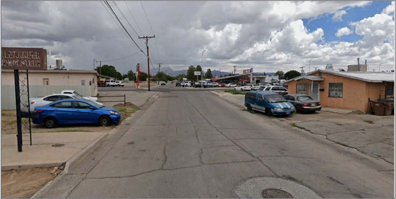
Image 14. Sidewalks are missing in multiple areas throughout the proposed MRA.
