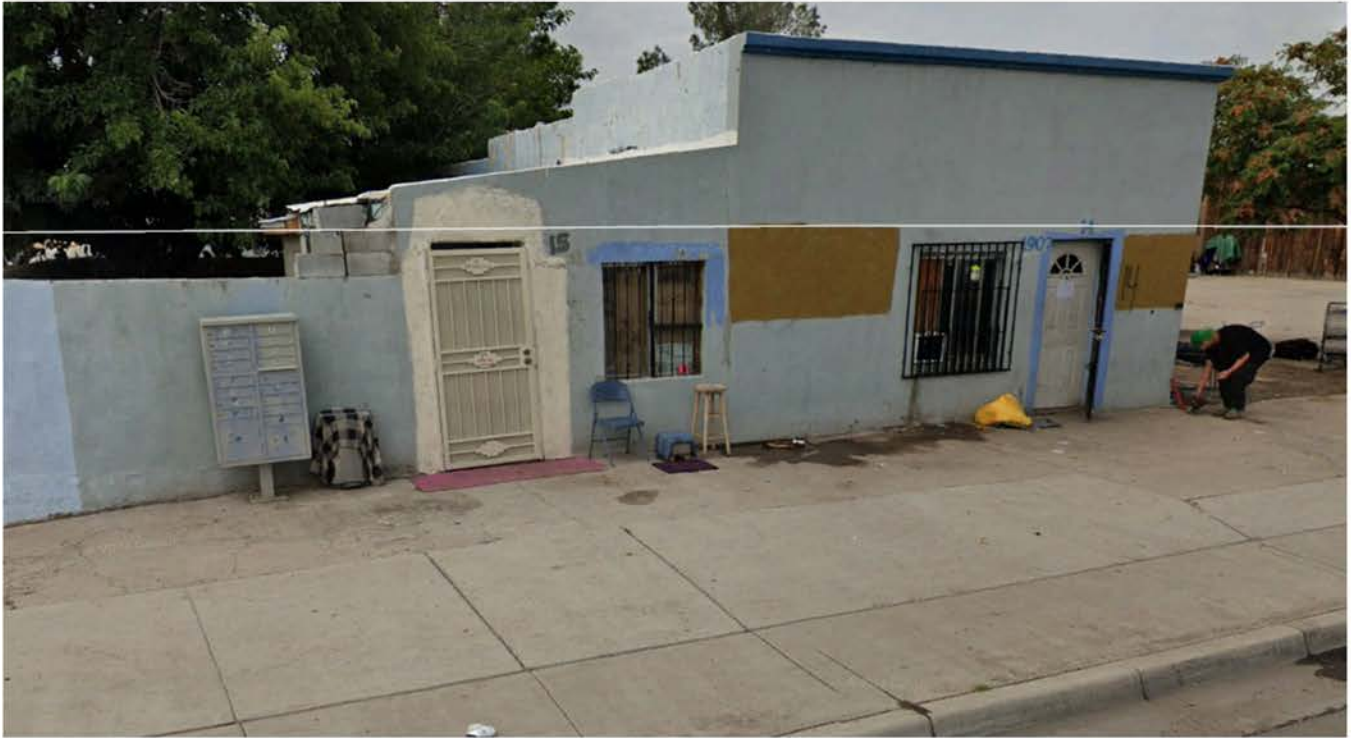
Image 24. Unmaintained housing unit in the West Picacho area
