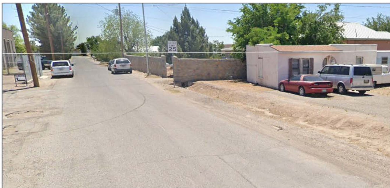
Image 23. Lack of sidewalks and deteriorated pavement adjacent to West Picacho Ave.
