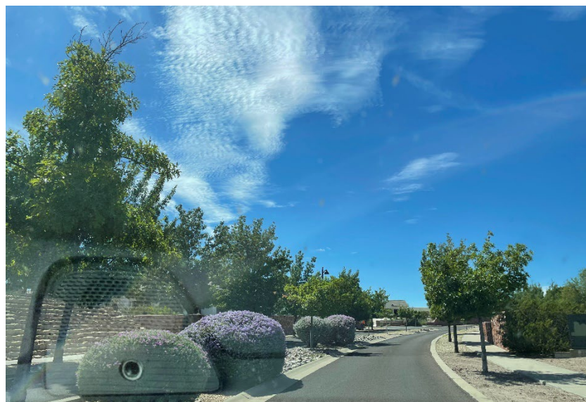
Figure 12. Morning Star Drive - Example Collector Road
