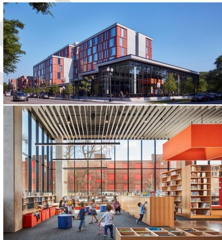
A public-private partnership of Chicago Housing Authority & Related Midwest. Little Italy Branch Library & Apartments, Chicago Public Library, Chicago, Illinois.
