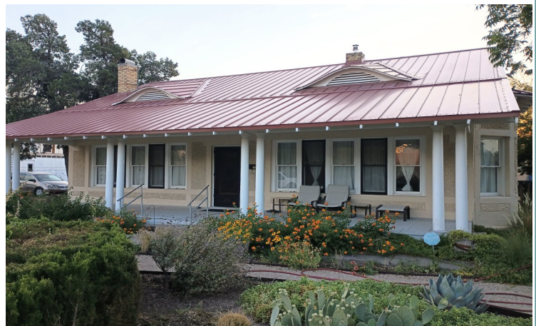
Eyebrow dormer (Alameda-Depot Historic District).
