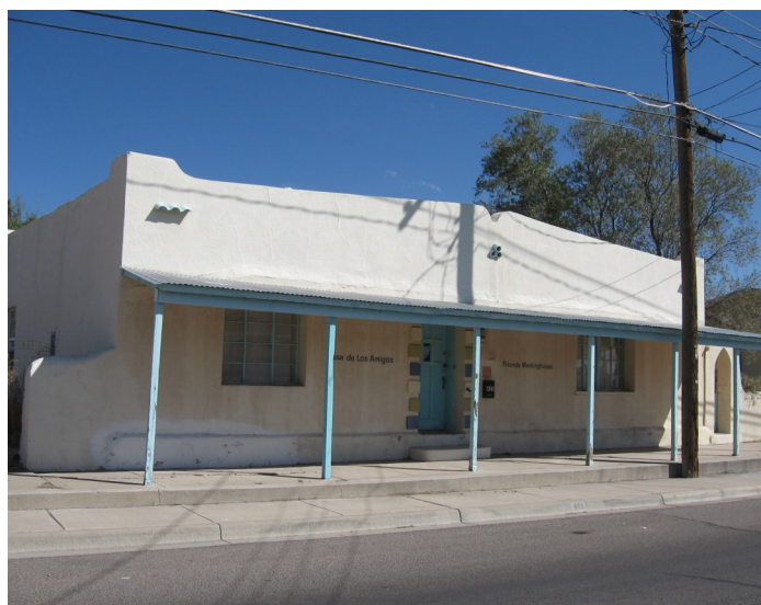
Southwest vernacular style building (Mesquite Street-Original Townsite Historic District).
