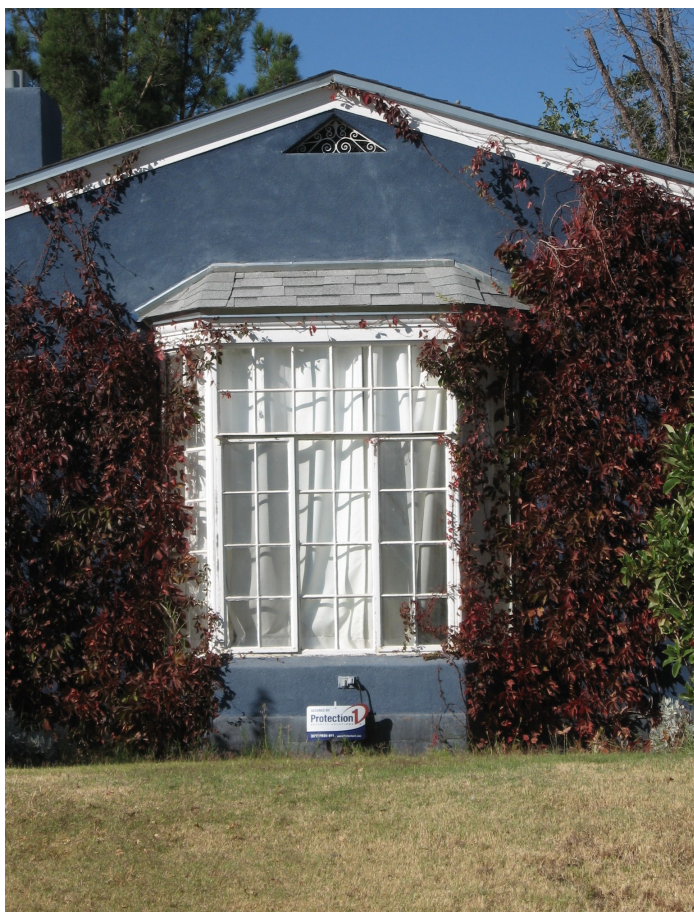
This bay window with eight-light casement windows helps define the Spanish Colonial Revival-style dwelling.
