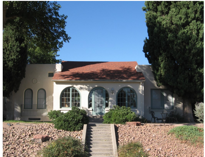
Spanish Colonial Revival style dwelling with arched window and door openings.
