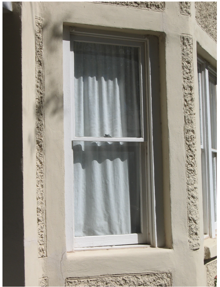
Preserve and maintain original wood sash windows (Alameda-Depot Historic District).
