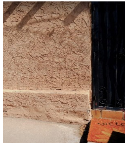
Many of the foundations in the historic districts are adobe covered with stucco. Stuccoed wall with foundation collar (Mesquite Original Townsite Historic District).
