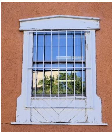
Security bars on a Territorial Style window. The 1/1 sash window is a metal-framed replacement for a larger original window.
