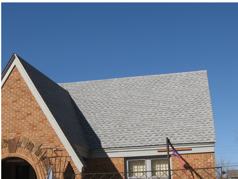
An example of a reflective roof on a historic dwelling is shown below.
