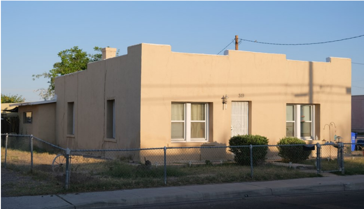
Southwest Vernacular with square parapets and double-hung windows (Mesquite Street-Original Townsite Historic District).
