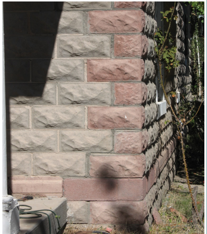
Rustic concrete block used as an exterior wall material on a number of dwellings during the early 1900s.
