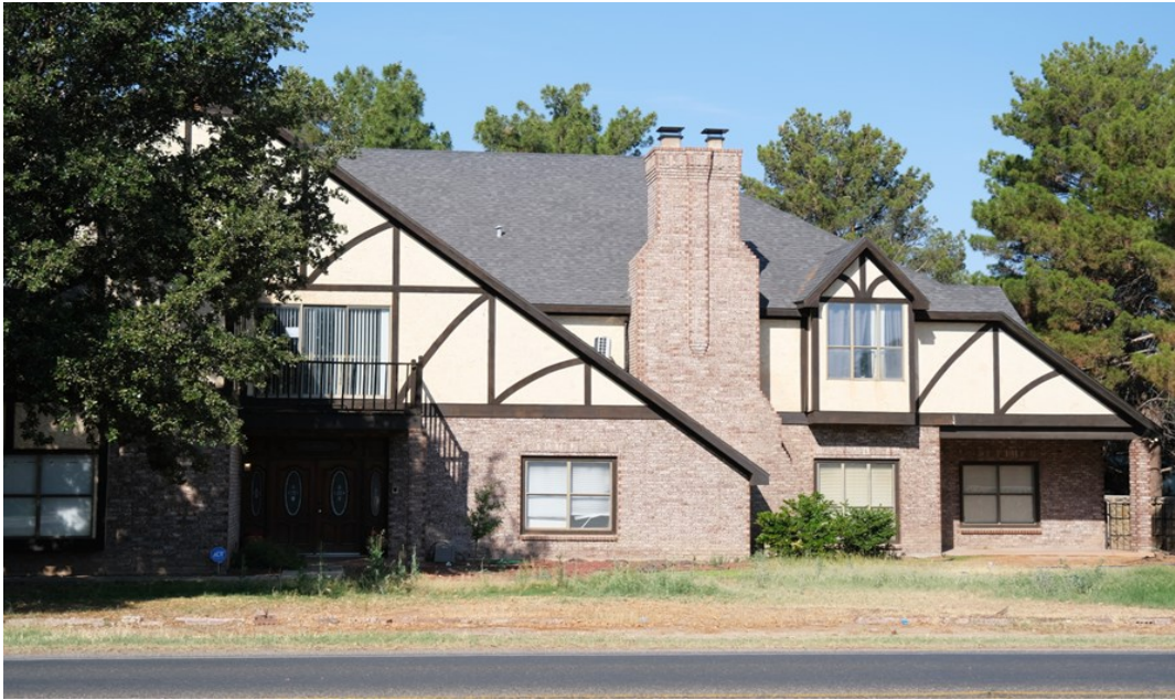
Tudor Revival Style with stepped chimney and faux half timbering.
