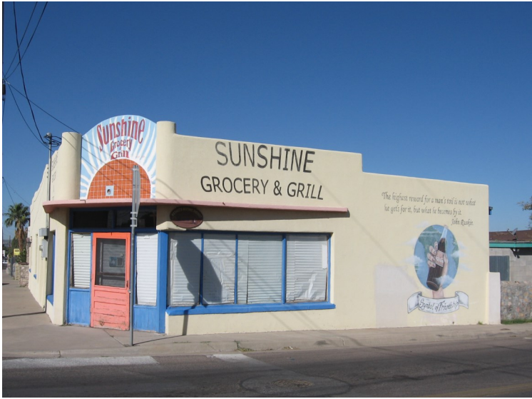
Vernacular commercial Art Deco (Mesquite Street-Original Townsite Historic District).
