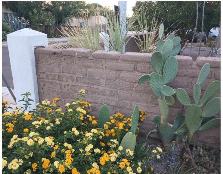
Stabilized adobe wall.
