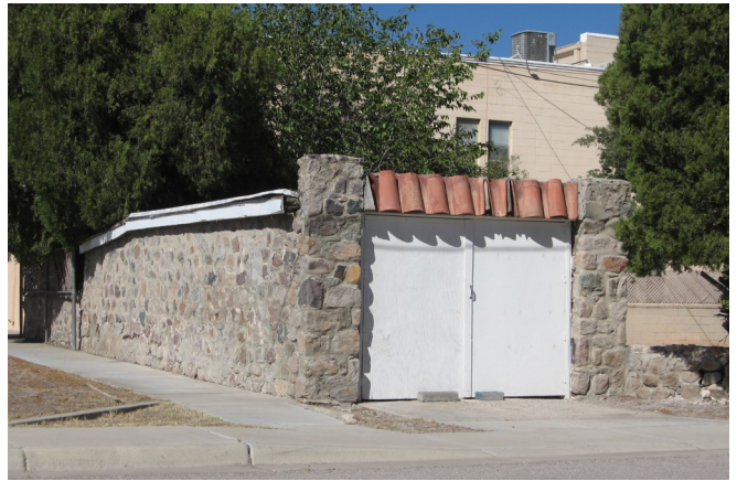
This stone garage retains much of its original design and character from the early 20th century.
