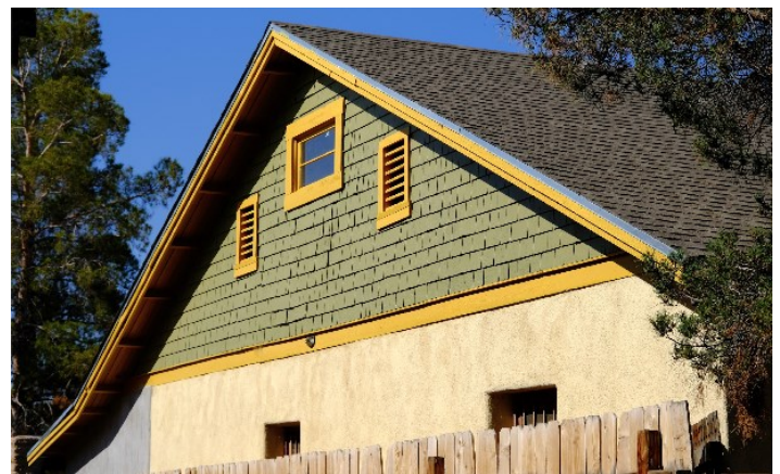
Original wooden shingles on vergeboard. Roof shingles have been replaced.
