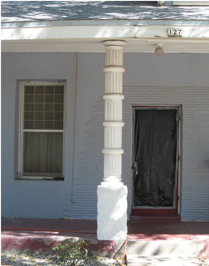
A few houses have unique porch columns made of cast concrete (Alameda-Depot Historic District).
