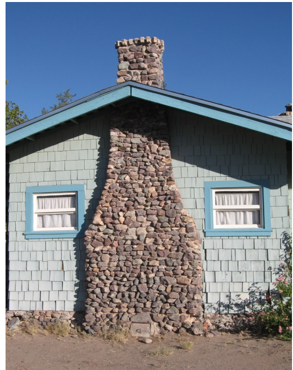
This cobblestone chimney is a significant aspect of this dwelling's architectural design and should not be altered (Alameda-Depot Historic District).
