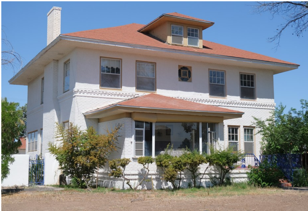
The symmetrical façade of this two-and-a-half story Hipped Box house was disrupted by a porch addition. First story walls are brick.
