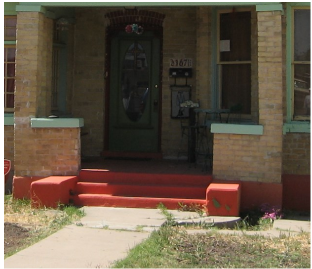
Preserve and repair as needed original concrete steps (Alameda-Depot Historic District).
