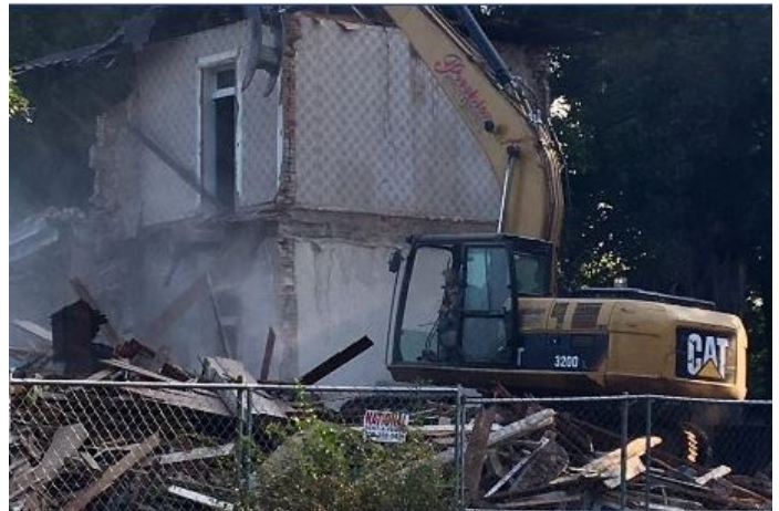
Demolition should always be the last option considered for historic buildings.
