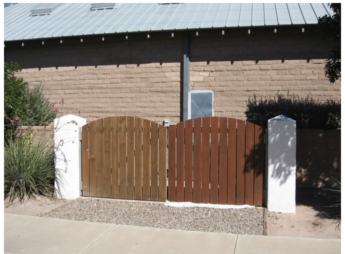
If mechanical units are placed on elevations visible from the street consider screening with landscaping, lattice, or fencing.
