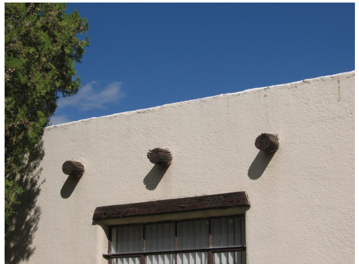
Vigas are protruding roof beams and are significant details of Pueblo Revival architecture. These should be preserved and not removed (Alameda-Depot Historic District).
