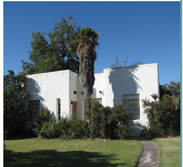
Historic neighborhoods appeal to new residents looking for unique architecture and quality of construction such as the Spanish-Pueblo Revival style house (Alameda-Depot Historic District).
