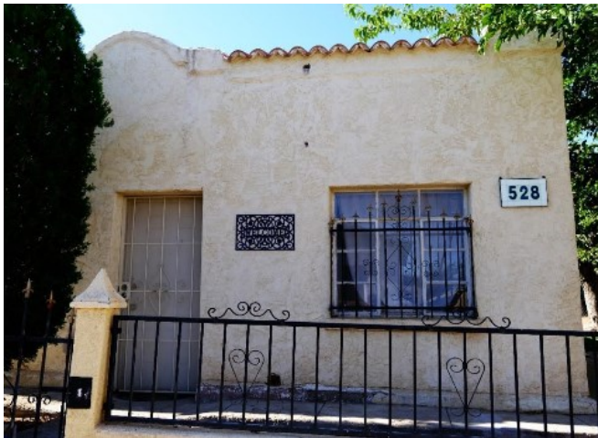
Use of decorative wrought iron as security bars on windows.
