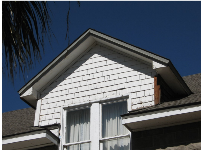
Preserve important roof features such as dormers on primary facades (Alameda-Depot Historic District).
