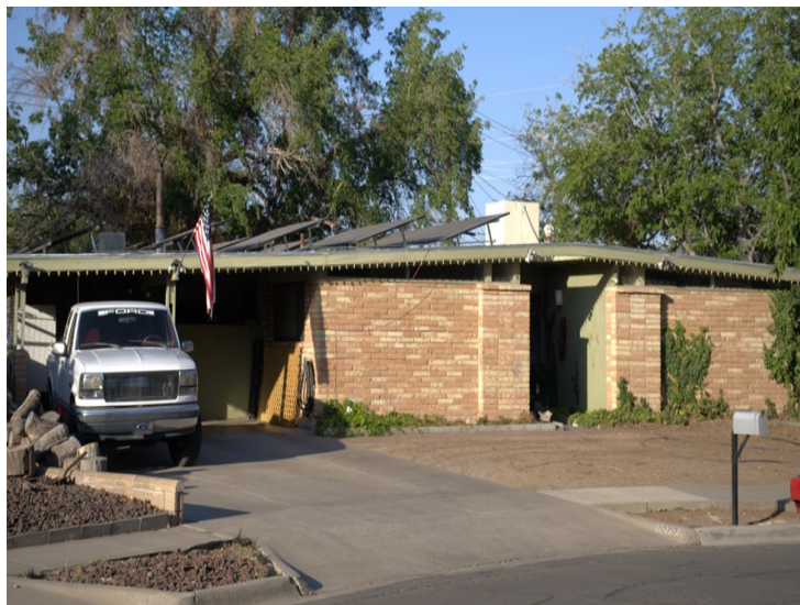
Mid-century Modern with recessed doorway and carport.
