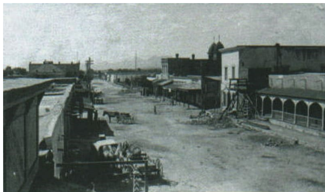
Main Street, ca. 1900, showing some of the early commercial buildings and the towers of St. Genevieve's Church (photo courtesy of Las Cruces Community Partners, LLC).
