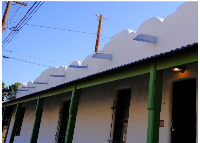
Metal canales above a corrugated metal, shed-roofed portal.
