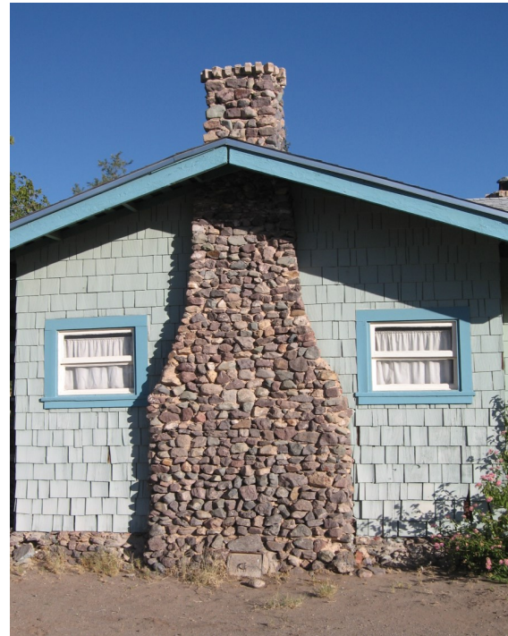
Wood shingle siding is a highly textured material that
