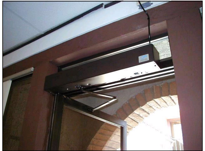
Original doors on commercial buildings can generally be retrofitted with push plates which activate door openers to allow wheelchair access.
