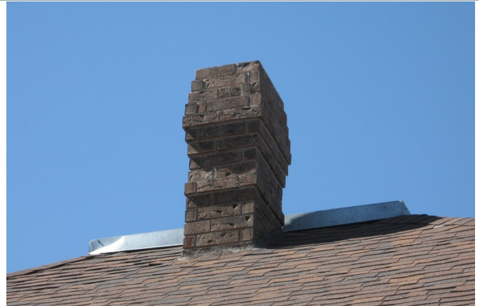
Corbelled brick chimneys at roof lines should be preserved and maintained (Alameda-Depot Historic District).
