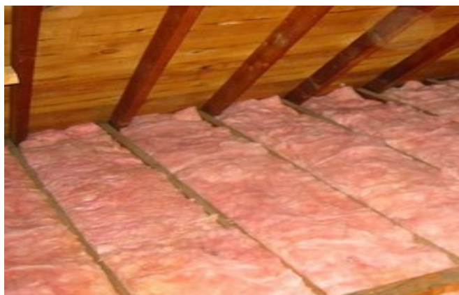
Adding insulation in ceilings is one of the most cost effective methods of saving energy in historic buildings.
