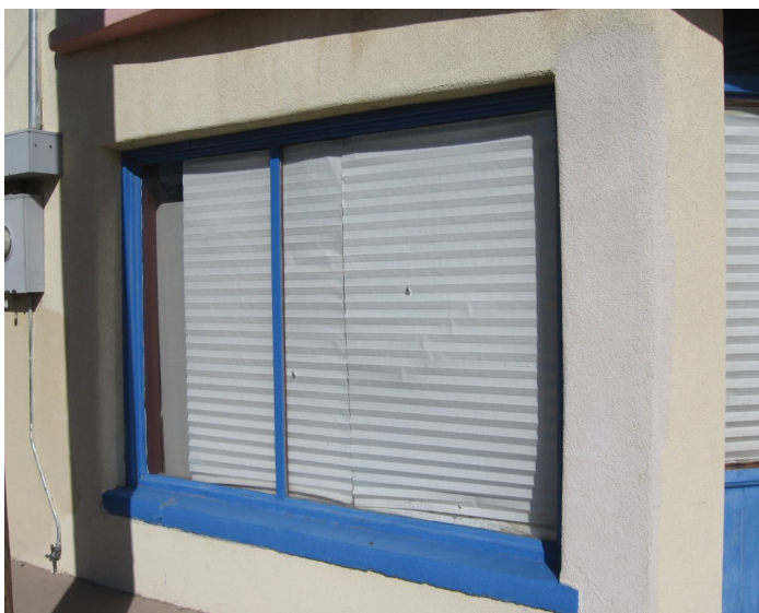
Preserve and maintain original steel or wood display windows (Mesquite Street-Original Townsite Historic District).
