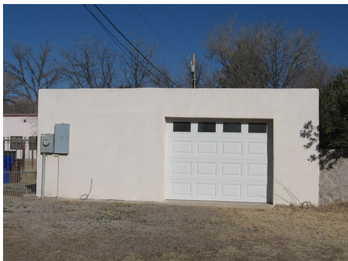
This new garage is located appropriately at the rear of the dwelling and reflects the main house's Pueblo Revival style.
