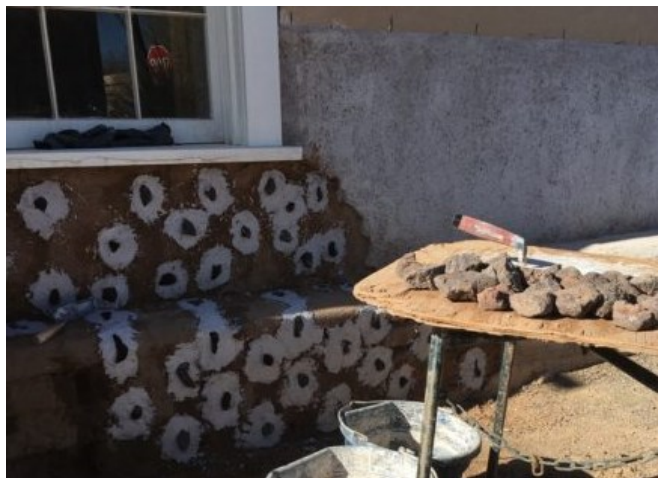
Correct adobe wall repair with requelas (small stone anchors) set in with lime plaster.
