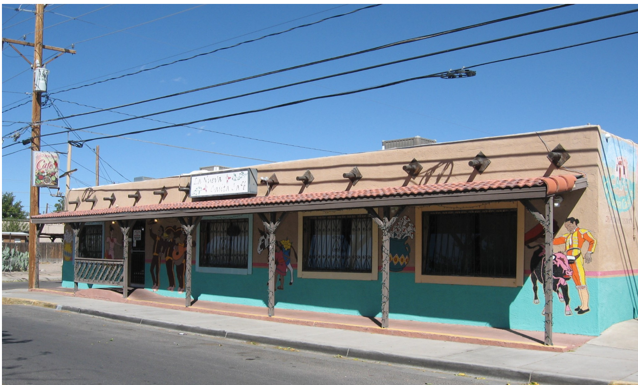
The commercial building at 195 N. Mesquite Street has an appropriate rebuilt portal with square wood posts and corbels (Mesquite Street-Original Townsite Historic District).
