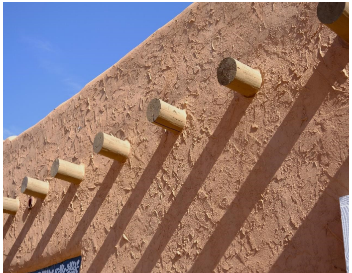
Exposed vigas (Mesquite Street-Original Townsite Historic District).
