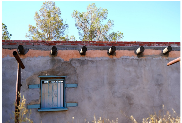
Exposed vigas with a brick coping on the roofline.
