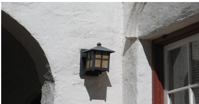
Appropriate replacement light fixture.
