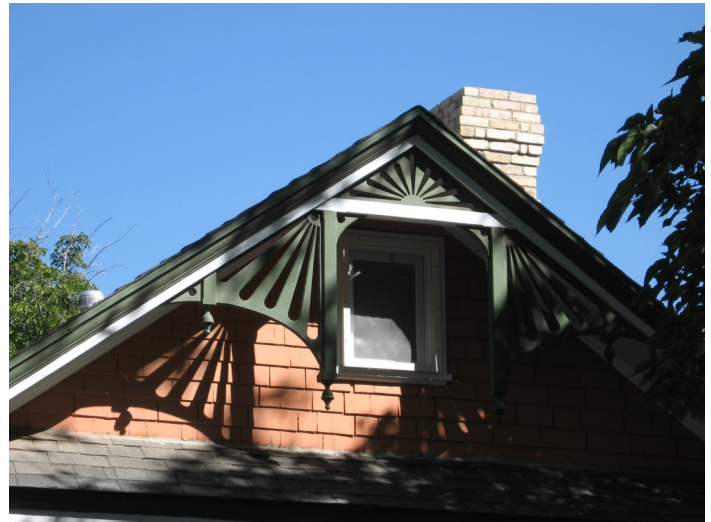
Woodwork trim like this gable detail provides texture and depth at the roofline and an opportunity for highlighting the woodwork through contrasting colors (Alameda-Depot Historic District).
