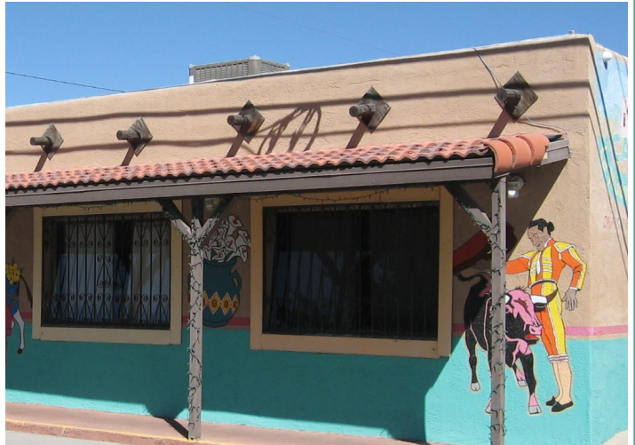
YES —Locate rooftop HVAC units back from the front wall to limit visibility (195 N. Mesquite Street).
