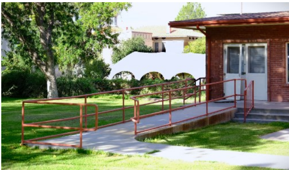
ADA ramp at the rear of this building (NMSU Campus).
