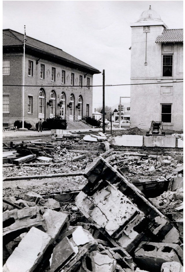
Demolished buildings at the corner of Main Street and Griggs Avenue in 1971 with the U.S. Post Office in the distance (Photo courtesy of the Special Collections Library, New Mexico State University).
