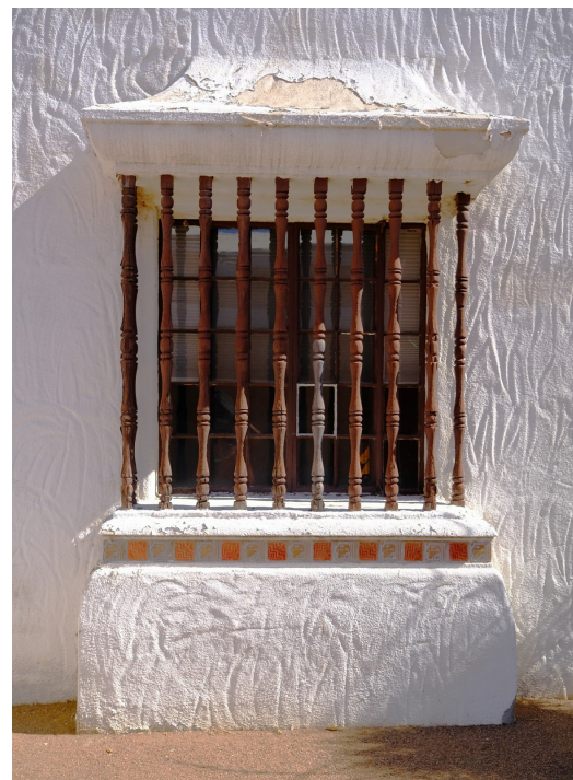
Use of turned wooded spindles as decorative security bars in an office window (Central Business District).
