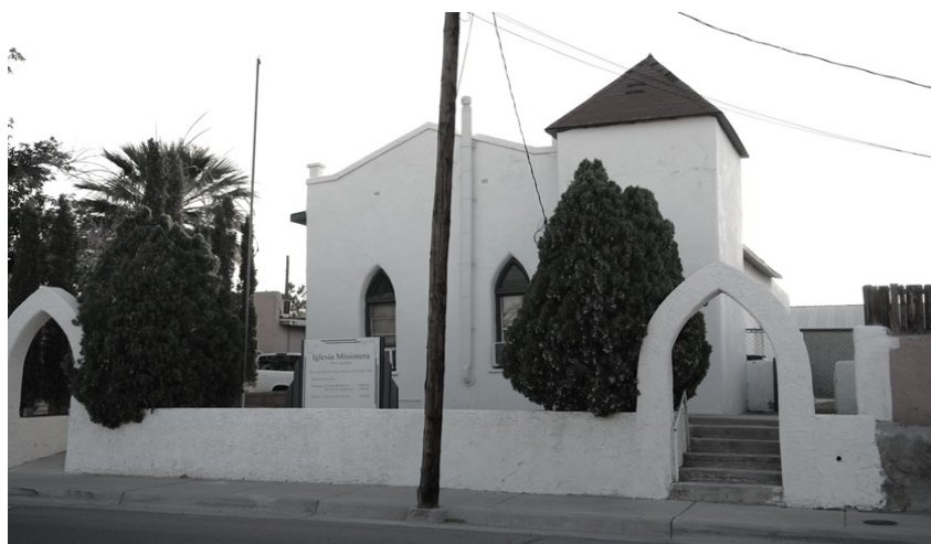
Iglesia Misionera. Vernacular Gothic Revival with Gothic arch window surrounds over square windows (Mesquite Street-Original Townsite Historic District).
