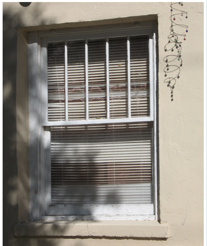
This five-over-one wood-sash window helps define the style and date of construction of the building (Mesquite Street-Original Townsite Historic Townsite).
