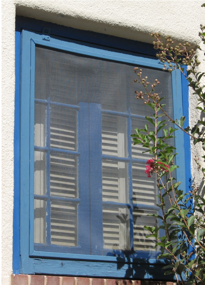
Preserve and maintain original screen panels (Alameda-Depot Historic District).
