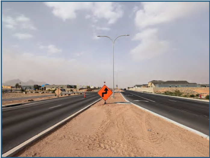
North view of Sonoma Ranch Boulevard
